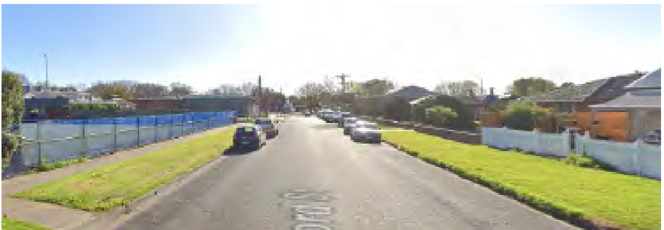
Google Street View along Lord Street
