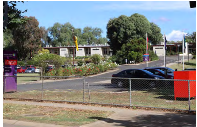
View west from Grant Street to Bacchus Marsh Hospital
