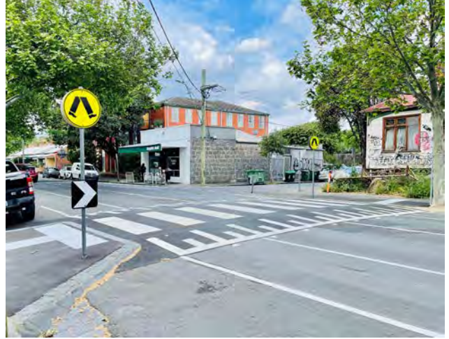
Raised pedestrian crossing to promote walking and pedestrian safety
