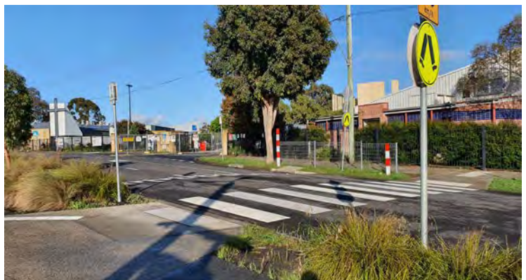
Raised pedestrian crossing, Middle Gorge Station
