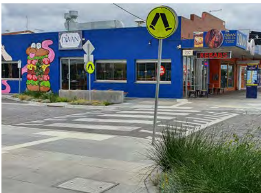
Raised pedestrian crossing, Thomastown
