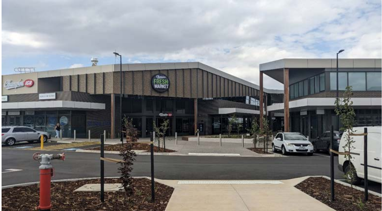
Figure 5-1: Maddingley Village – a new small neighbourhood centre, with a mix of street-facing and internal spaces as well as a variety of retail and non-retail activity, with medium density housing clustered nearby.
