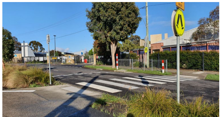
Raised pedestrian crossing, Middle Gorge Station
