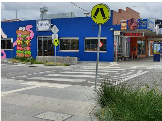
Raised pedestrian crossing, Thomastown
