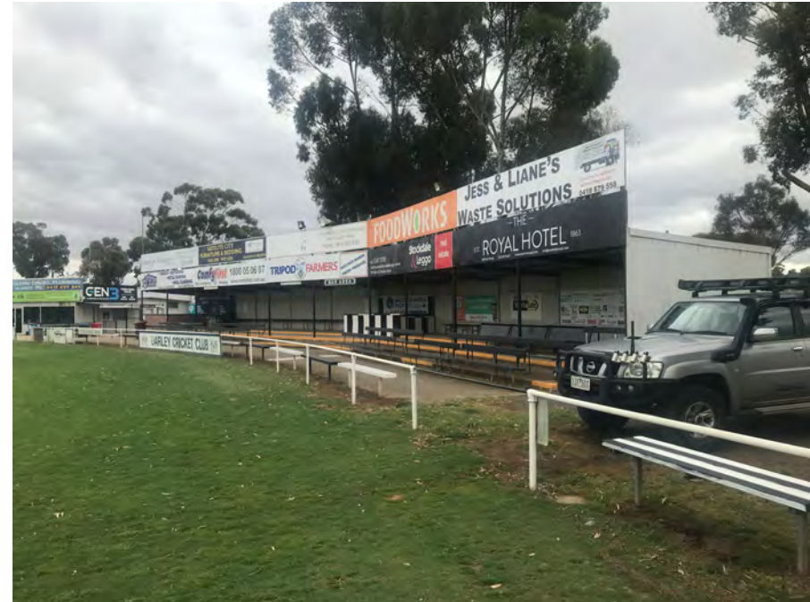
Figure 1. Grandstand on western side of Darley oval
