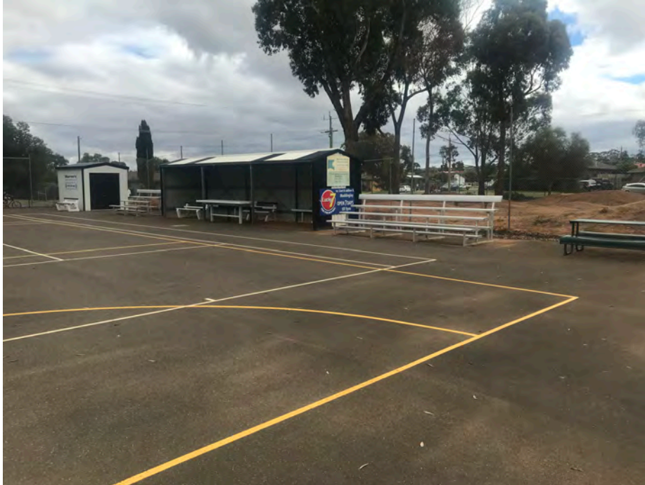
Figure 1. Netball/tennis courts (pre 2021 upgrade) and shelter
