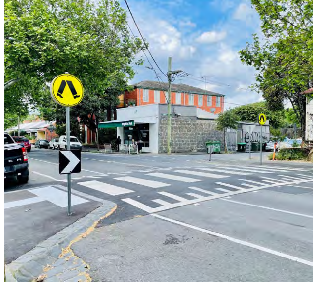
Raised pedestrian crossing to promote walking and pedestrian safety
