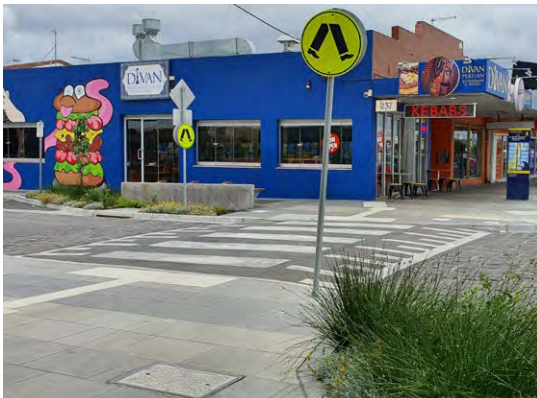
Raised pedestrian crossing, Thomastown
