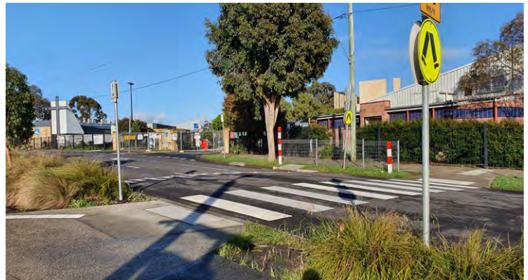
Raised pedestrian crossing, Middle Gorge Station
