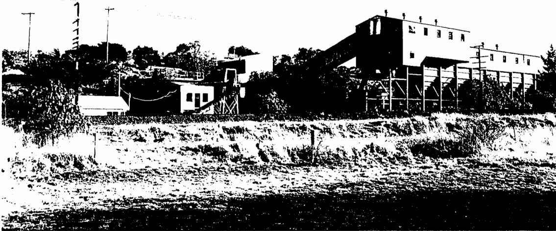
COAL LOADING BUILDING.
