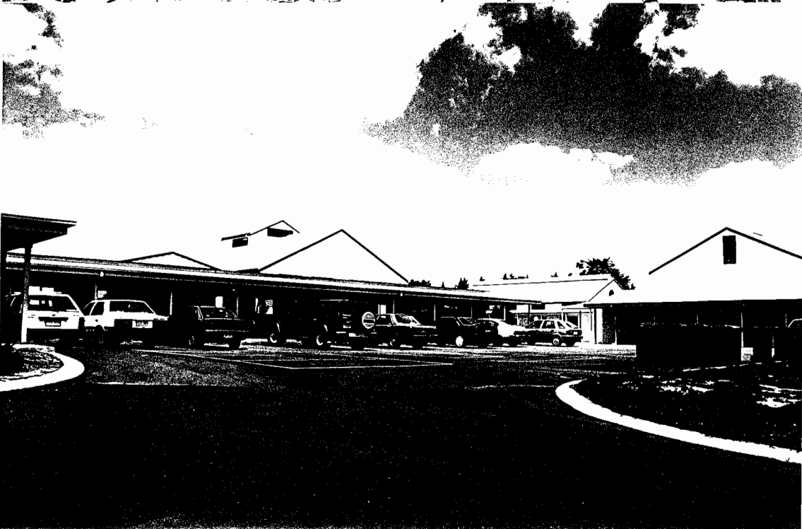
FORMER MINE BUILDINGS AT BACCHUS MARSH GRAMMAR SCHOOL.
