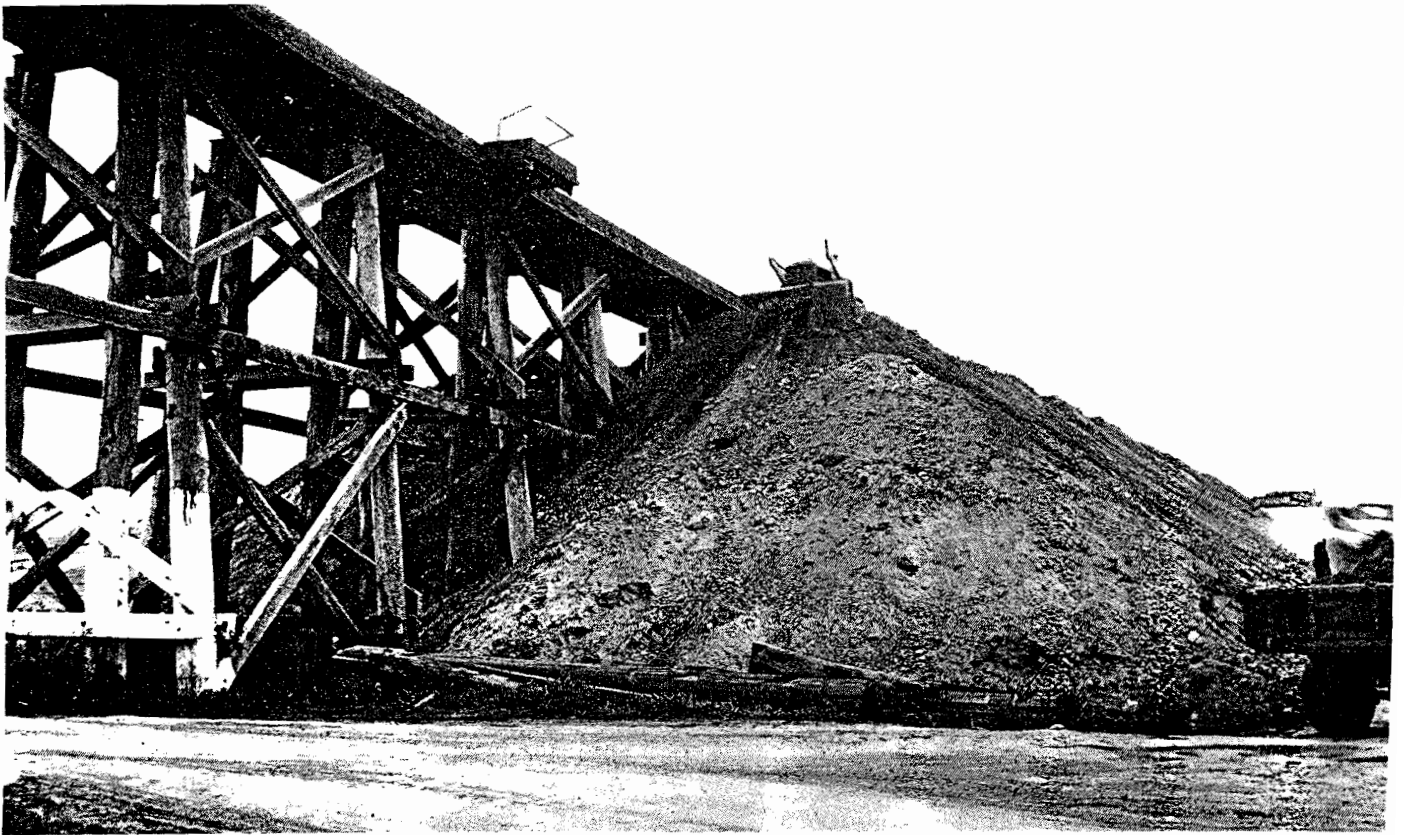
FORMER TIMBER BRIDGE & COAL MINE OVERBORDEN AS EMBANKMENT, 1922 MURRE & COMES
