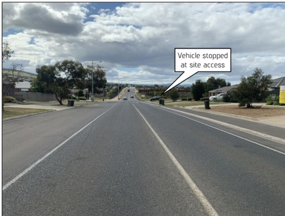
Figure 5 Southern site distance check (83m)
