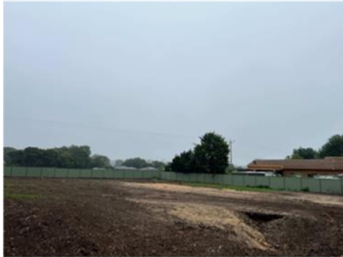
NORTH WEST VIEW
