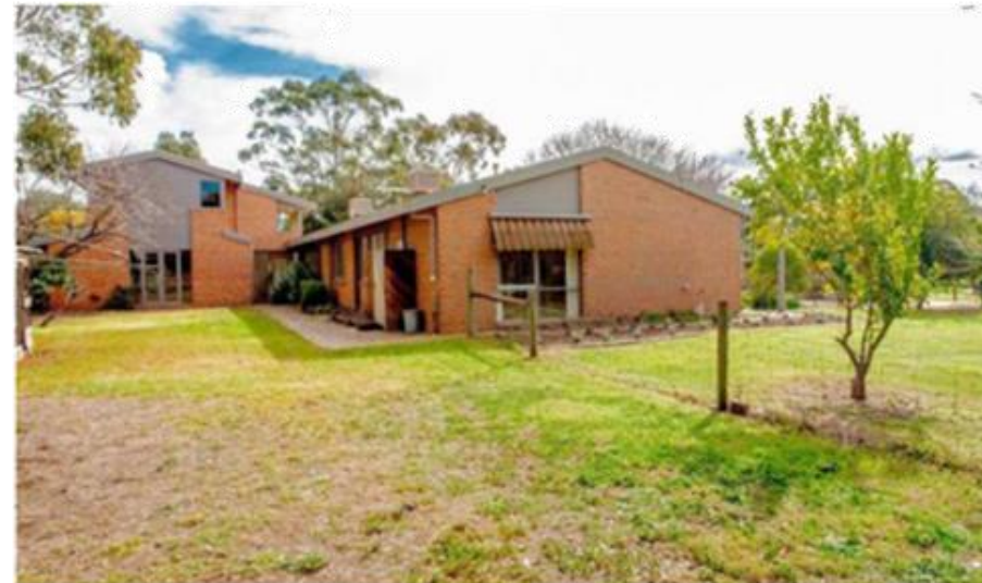
#84 ELLERSLIE COURT - ADJACENT TWO STOREY BRICK VENEER DWELLING
