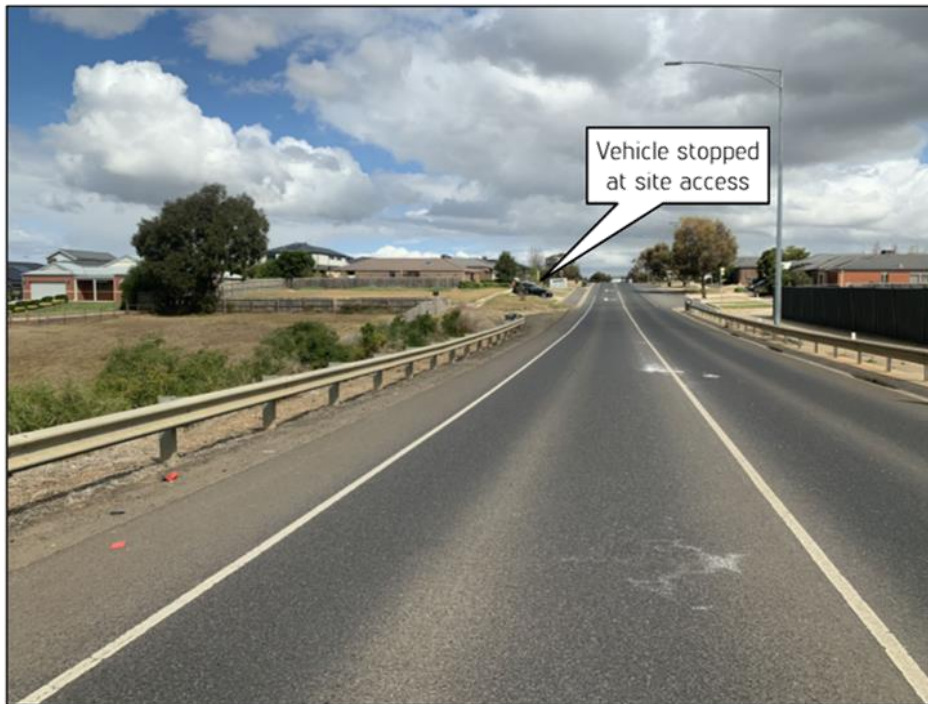
Figure 4 Northern site distance check (83m)
