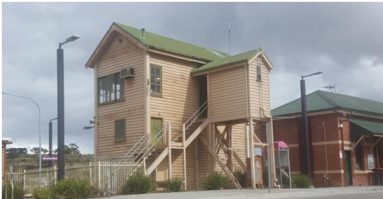
Figure 3: View of the Signal Box looking to the south-west
