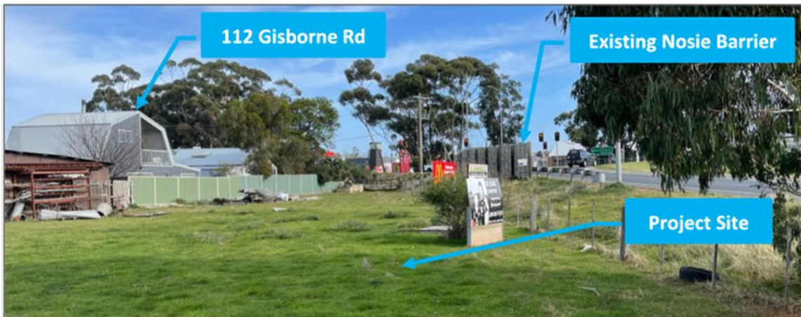
Figure 5 Existing Noise Barrier
