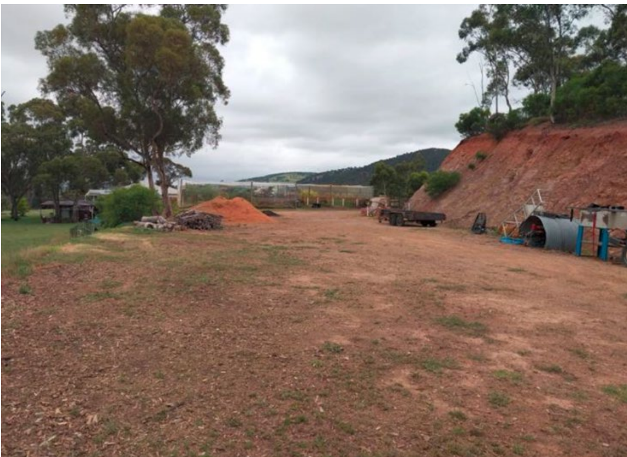
Figure 3: Existing earthworks area
