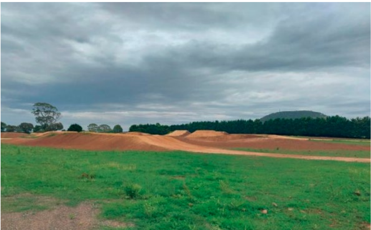
Figure 4: View of the completed track
