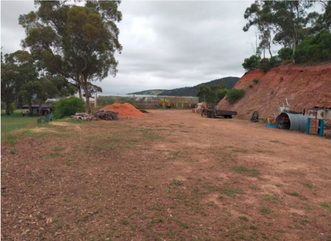
Figure 3: Existing earthworks area
